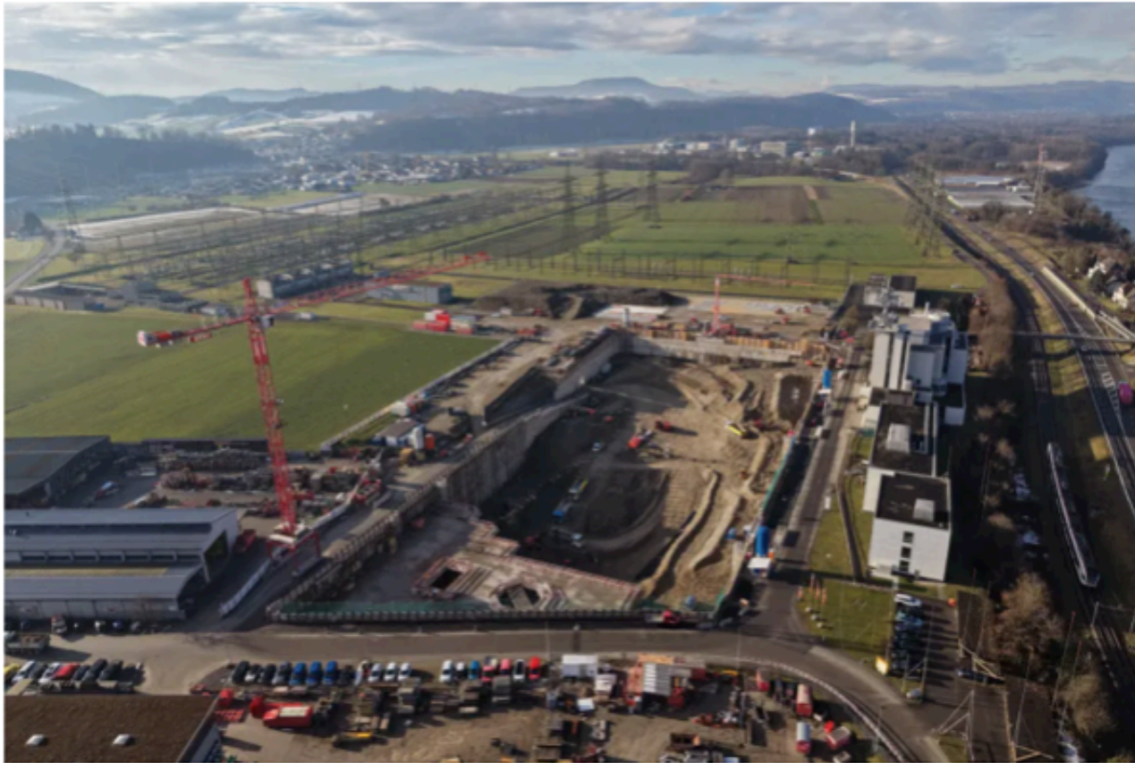
▲ An aerial view of the ongoing construction work on the world's largest redox-flow battery storage system in Laufenburg, canton Aargau. Flexbase
